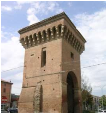
Fig.13. One of the gates with the residual presence of the wall
