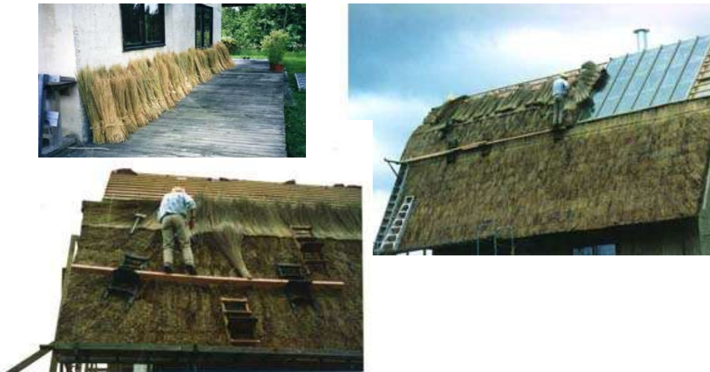
Fig. 9 Thatching roof with bulrush
