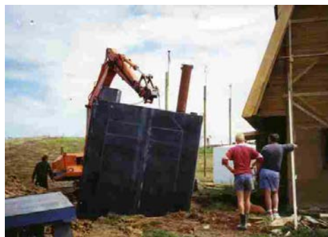
Fig. 1. Ozeki septic tank to change any organic inputs into bio-gas
