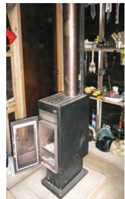
Fig.6 Solar panels in the above and the wet back in the shed to make hot water
