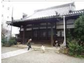
Fig. 3. Outward appearance of JYOSHINJI temple, Nagoya, Japan
