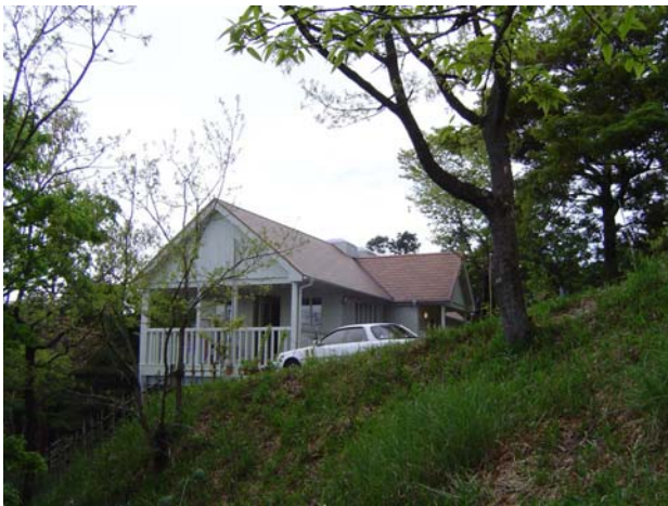
Photo 10. Exterior view of east side of house.
