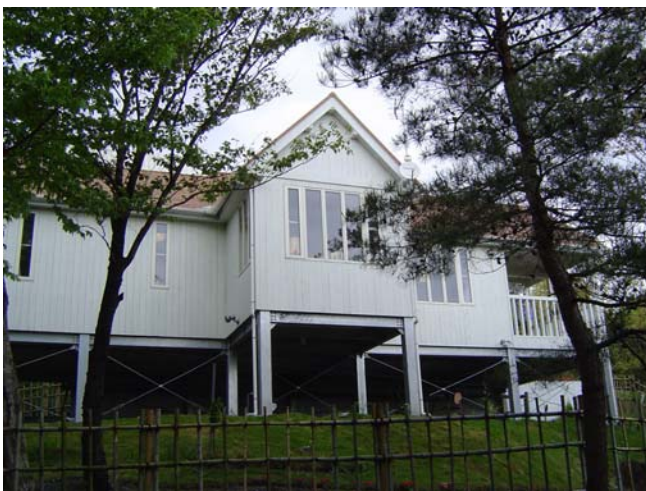
Photo 2. Exterior view of rear of house.
