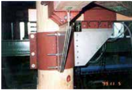
Fig. 13. Installed damper at lower Nuki.
